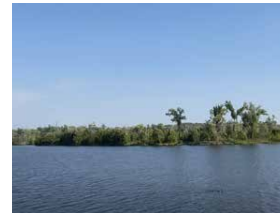
View from the top of 1st Street berm
