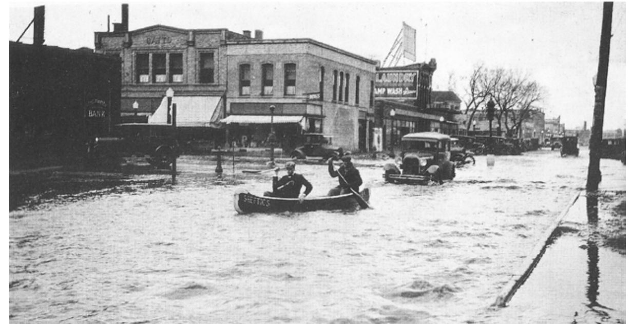
1929 FLOOD, 1ST AND 3RD AVENUE
